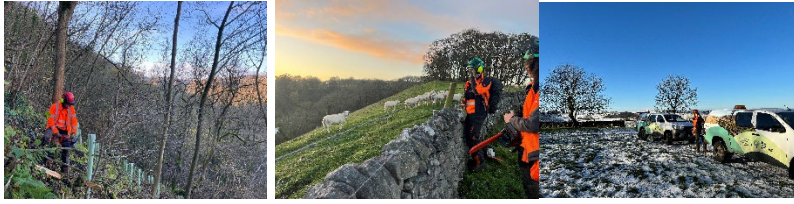
Photos by Natural England: Working on site
